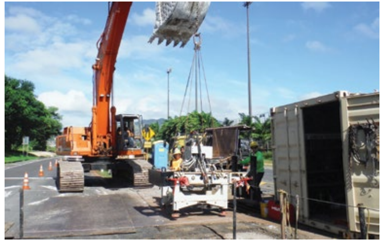
Figure 7. Jacking shaft set-up
