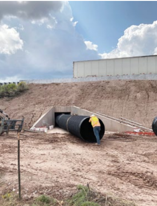
The pipe was easily pushed into place using skid rails
