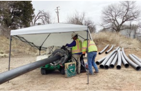
Pipe Fusion of 8-Inch HDPE
