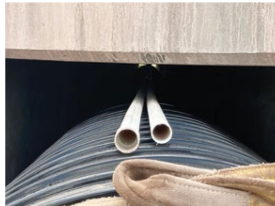
Grouting required two days
