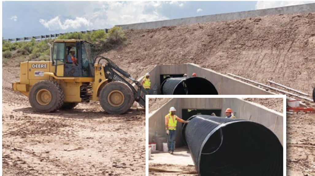
Twelve 30-foot-length segments totaling 360 LF were pushed into the existing culvert
