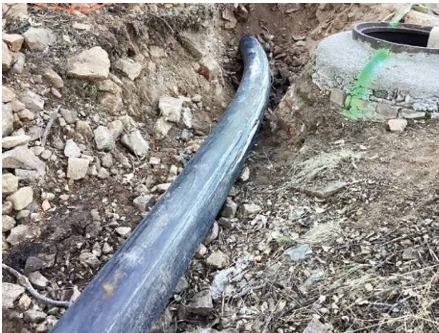
Insertion Pit for 8-Inch HDPE pipe
