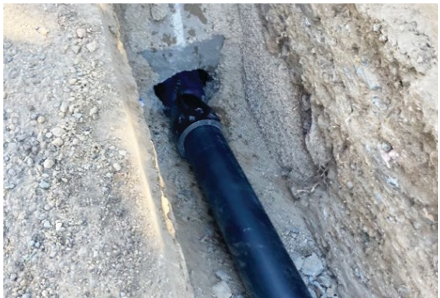
Bursting Head with 8-Inch HDPE Pipe
