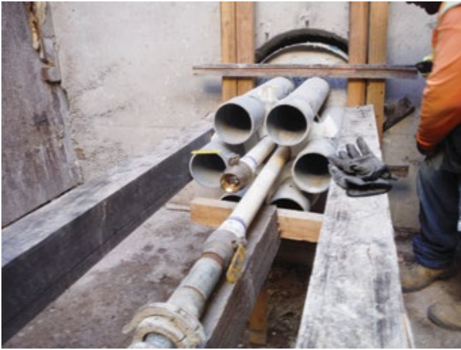
Figure 10. Conduit setup inside casing pipe with bulkhead
