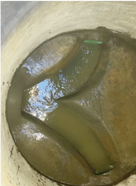
MH Invert Rehabilitation after burst
