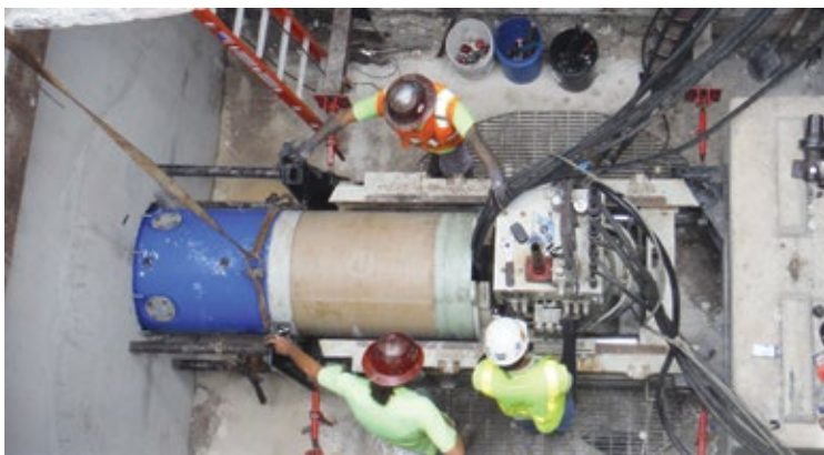
Figure 8. Powered cutterhead with GFR casing pipe
