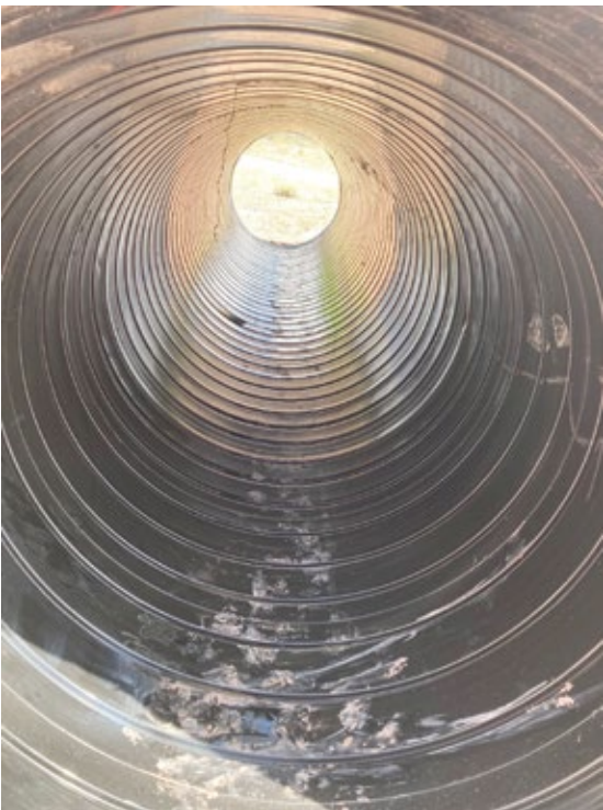
Unique spiral rib profile of the pipe met the hydraulic requirements for the project
