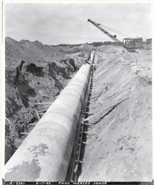
Park Merced Sewer 1942
