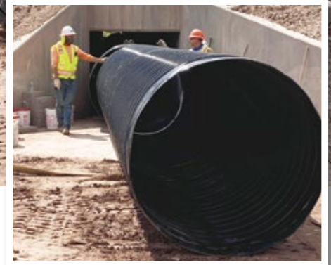
Twelve 30-foot-length segments totaling 360 LF were pushed into the existing culvert
