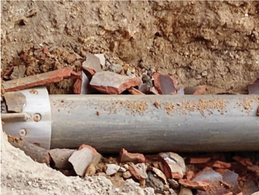
Bursting old VCP with new HDPE
