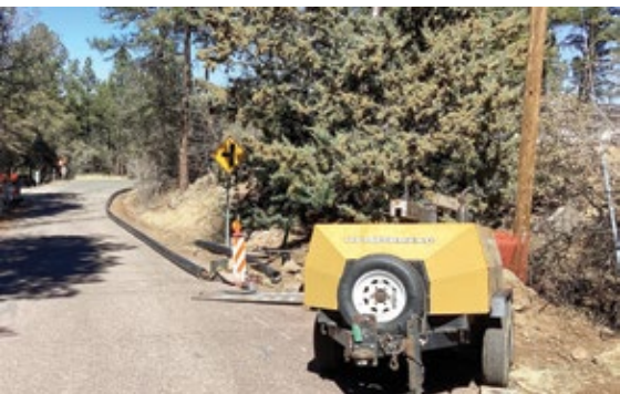
Typical Winch Set Up
