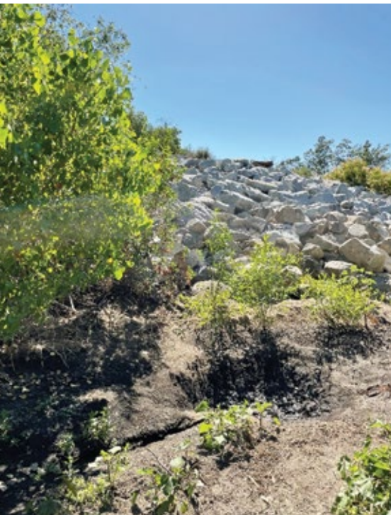
Figure 6 – Existing Streambed Stabilization
