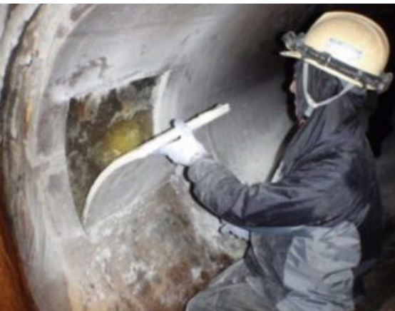
Figure 1: Sampling of the Original Installation of CIPP
