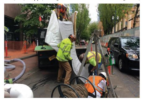
Figure 2: Inserting 10-in. UV CIPP liner on SW Yamhill St. located underneath railroad tracks.
