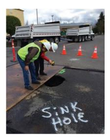
Figure 1: Sink hole over failed 42in. sewer requiring a quick repair
