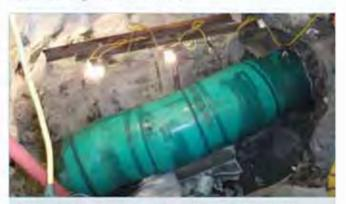
Figure 4: The completed 36-in. diameter product pipe inside the frozen soil cavity.
