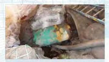
Figure 3: Initial cavity around the product pipe (green) and casing prior to removal of the pull head and installation of the insulated tarps. Note the frost development on the back and upper face of the cavity.
