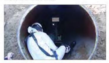
The electromagnetic inspection identified 58 pipe sections with electromagnetic anomalies out of approximately 10,000 pipes inspected, a distress rate of 0.6 percent (industry average is 4 percent). This project provides an example of how utilities can manage aging infrastructure while working within a tight capital budget, effectively extending the useful life of the asset. The project was awarded an honorable mention in Trenchless Technology magazine's Project of the Year awards.
