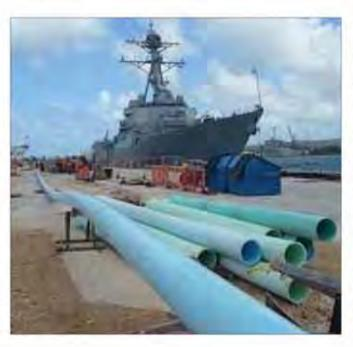
Fusible PVC pipe is now regularly designed and installed in Hawaii Department of Transportation (HDOT) right-of-ways (airports, harbors, and highways), under major roadways, including H3, Kamehameha Highway and beneath Dillingham Airfield.
