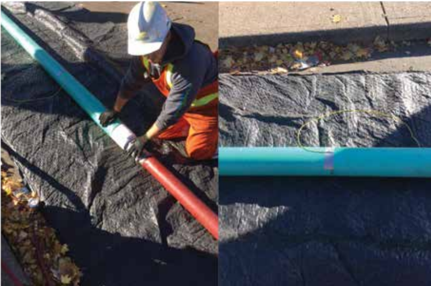
Figure 2: Lateral sample creation on site with thermocouple for temperature monitoring
