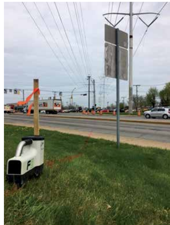
Large overhead powerlines, various buried utilities and traffic light sensors were the primary causes of heavy interference
