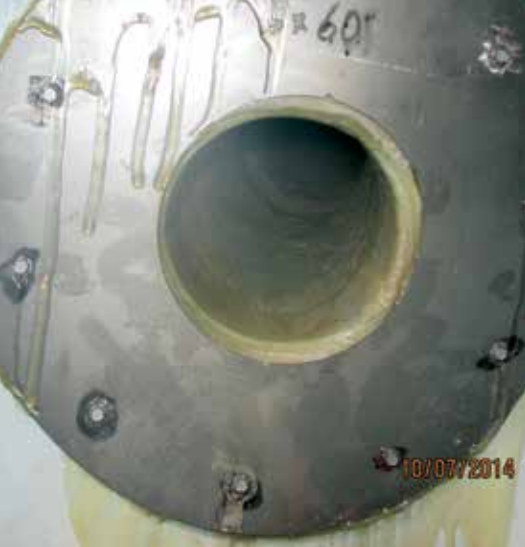
The End Result: A one-piece structural lateral lining and sealed connection to the main
