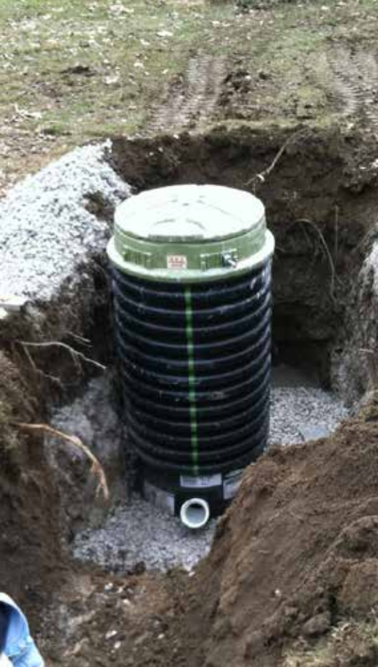
New grinder pump in place
