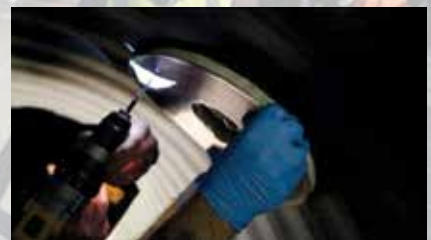
Anchor installation onto the brim through the steel ring
