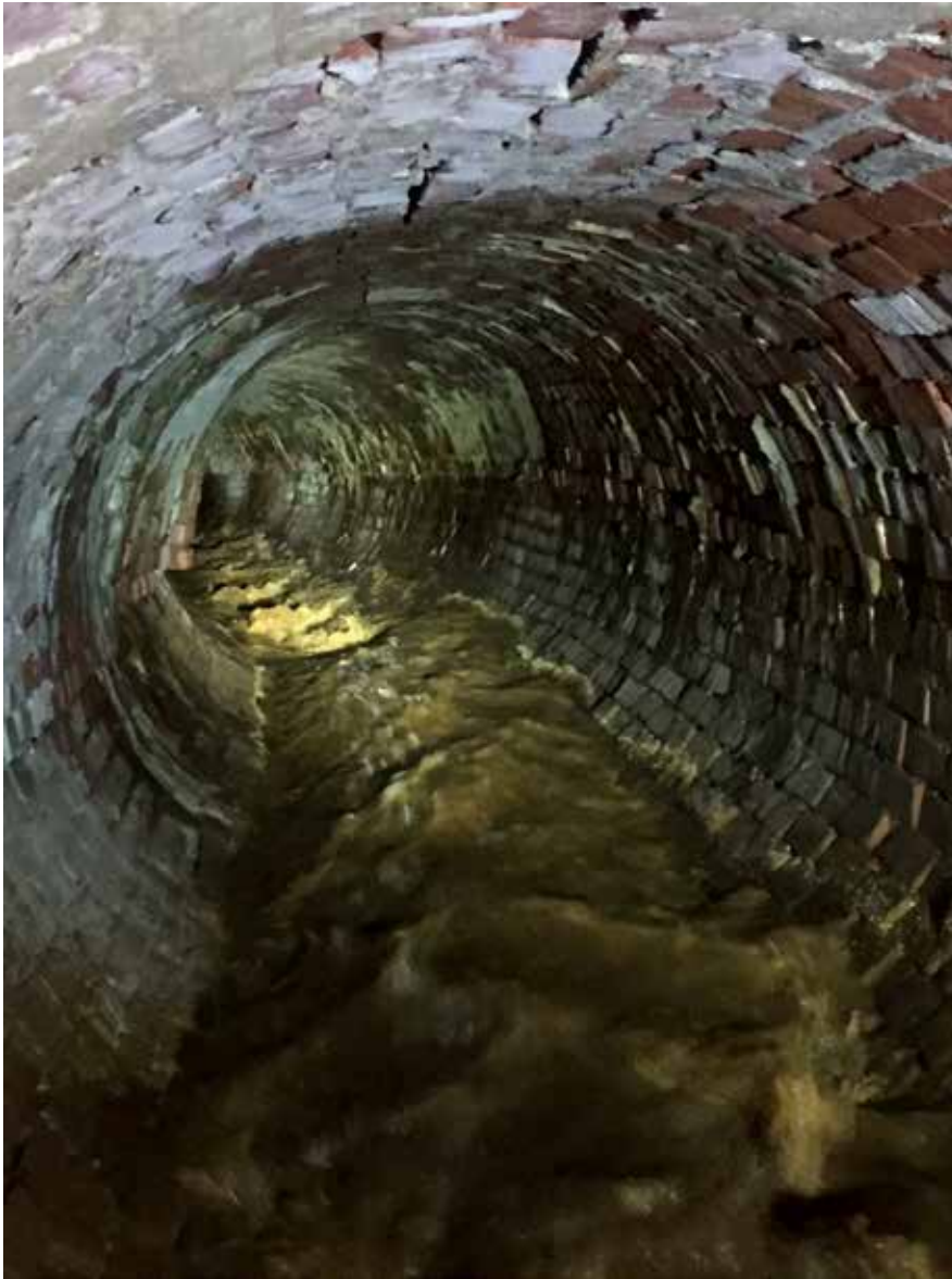
Original brick sewer showing curved section
