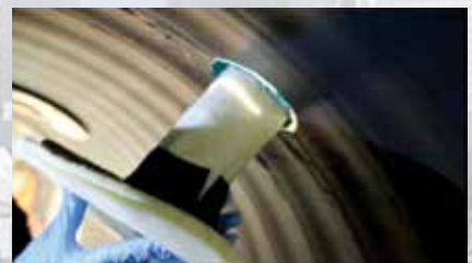
Lapel Liner inserted into service line
