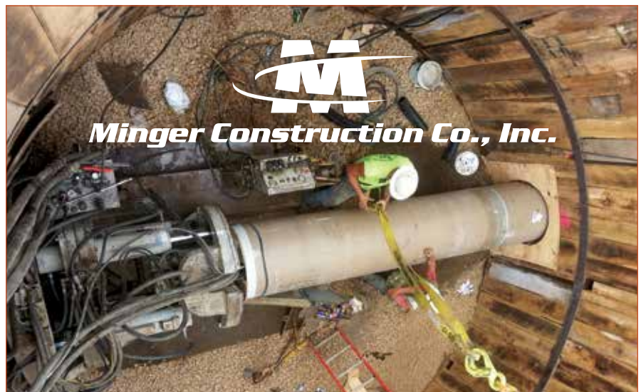
Tight working conditions in active urban areas make trenchless installation using the Pilot Tube Method the best option.
