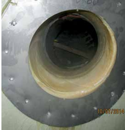
The End Result: A one-piece structural lateral lining and sealed connection to the main
