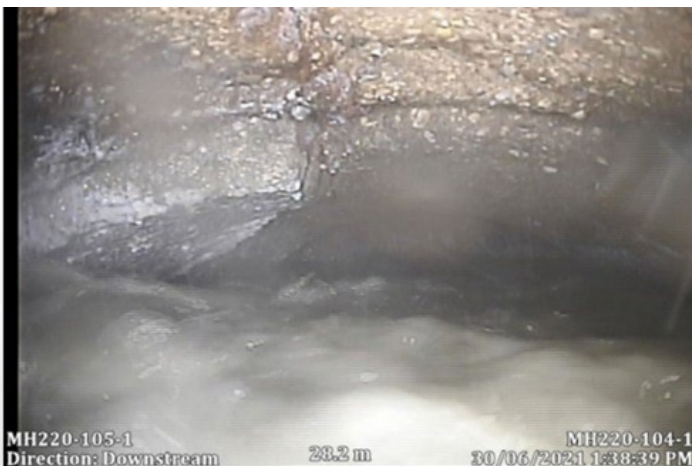
Figure 9 - HCI Severe fractures and Settlement Related Defects at MH Structure
