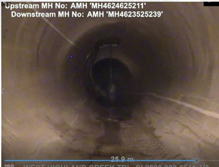
Figure 15. HCI Completed CIPP through Severe Fracture
