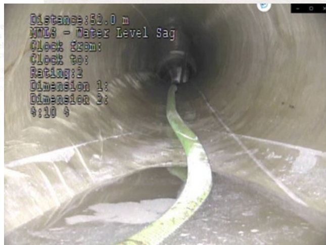
Figure 14. EDTS – Completed CIPP Liner through Settled Portion of Trunk Sewer
