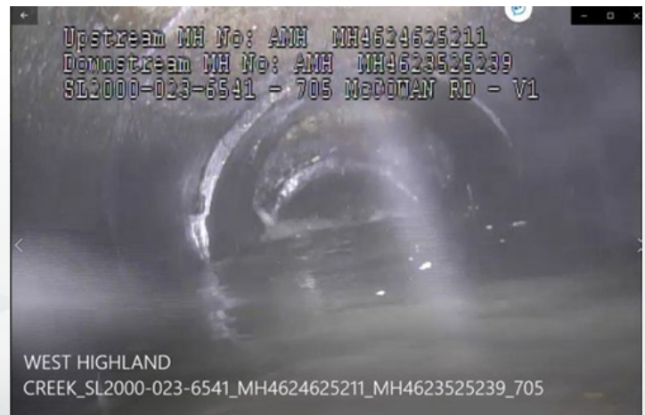
Figure 9 - HCI Severe fractures and Settlement Related Defects at MH Structure
