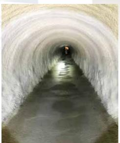
Figure 10. Completed lining of the original 96 x 96-inch brick/granite arch tunnel
