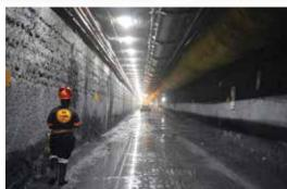
The MDM5000 is particularly useful wherever a rectangular profile is needed, such as train tunnels requiring a flat invert. The rectangular profile requires 30% less rock to be removed as compared with a circular cross section. Photo CREDIT: FRESNILLO PLC
