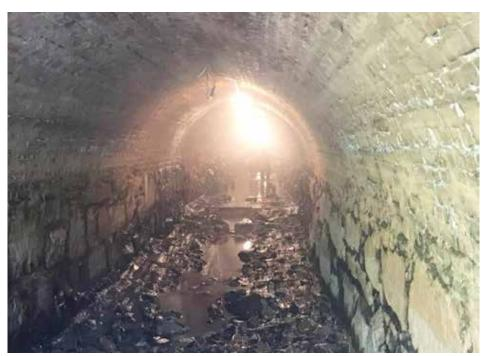
Figure 1. Internal view of the existing granite and brick tunnel prior to rehabilitation
