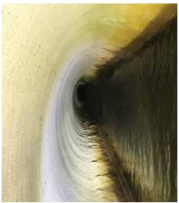
Figure 12. View of the completed lining at the outlet of the tunnel at the Broad River after 2 years of Service
