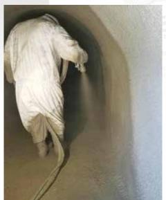
Figure 9. Hand spray application of the geopolymer lining
