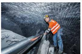
Robbins Field Service personnel inspect the cutting face of the MDM5000 tunnel operation. To date, the machine has bored more than 1,700 m at rates up to 52 m in one week and 191 m in one month.
