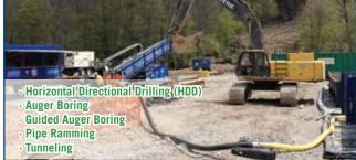
Diameters up to 48 inches and distances over 7,500 LF through dirt and rock. Atlas' fleet of drill rigs have the capabilities of up to 100,000 to 750,000 lbs. of drilling thrust/pullback force.
