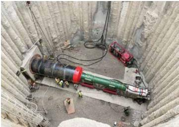
Photo 1 - Pipe ram equipment using a hydraulic hammer to install an 84-inch steel casing on the Willamette Water Supply Program Raw Water Facilities project in Wilsonville, Oregon
