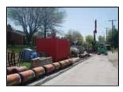
The Shively Interceptor Project in Shively, Ky., is the third largest pilot-tube microtunneling (PTM) project ever completed in the United States. Midwest Mole was the contractor on the project that consisted of the installation of more than 10,678 lf of vitrified clay pipe (VCP)
