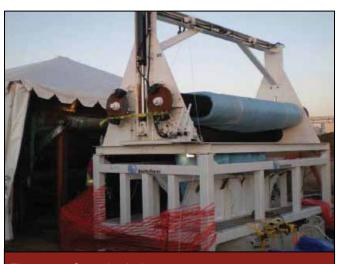
Figure 3 - Over-the-hole wet out.
