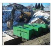
Insituform Technologies Inc. was the contractor on the Saskatoon Interceptor Trunk Sewer Rehabilitation project, which included the cleaning and CIPP lining of 1,007 ft of 84-in. reinforced concrete pipe. The project was completed with the largest sanitary sewer bypass pumping project in Western Canada.
