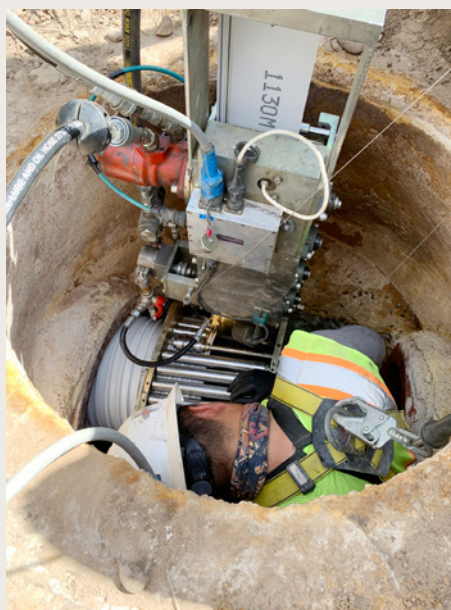
Winding machine is positioned at the base of the manhole
