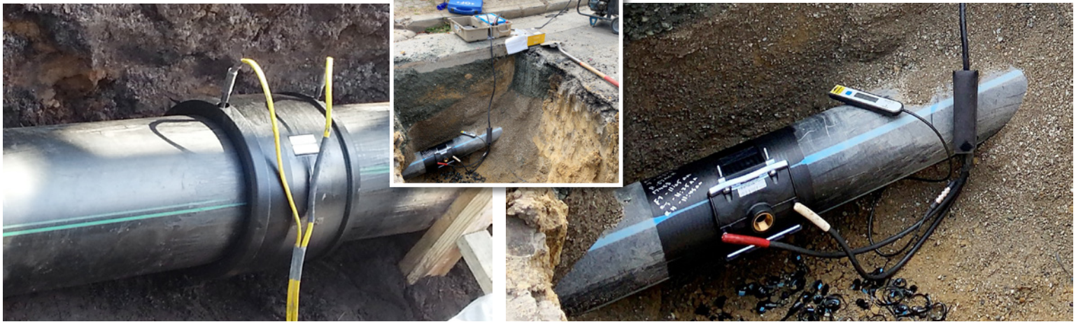
Electrofusion in Pit
