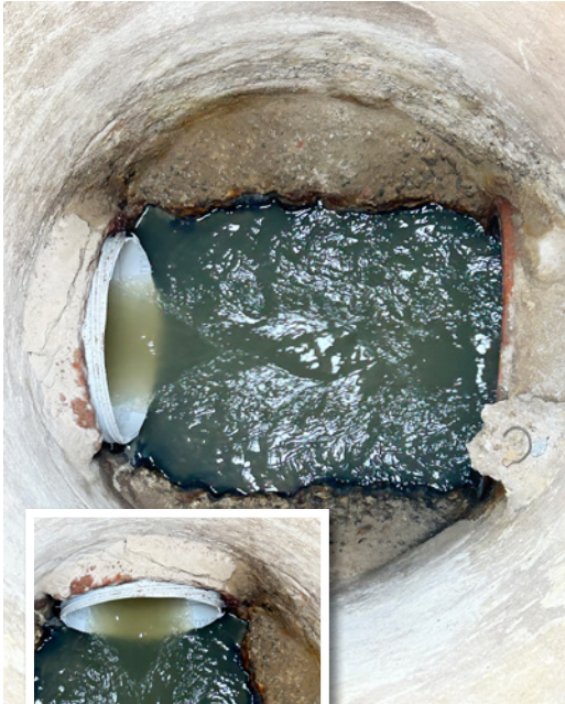
Liner is installed from the downstream to the upstream manhole
