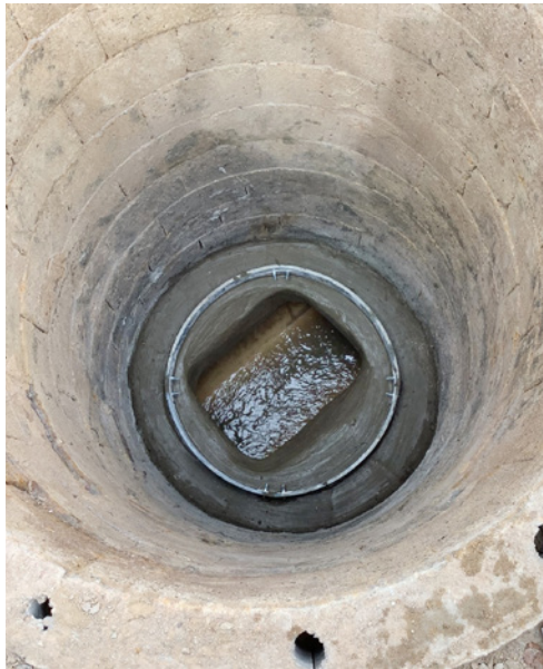
Form for manhole grout ring
