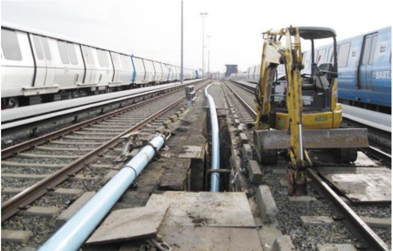
Trenchless methods overcame extreme challenges of space and rail proximity
