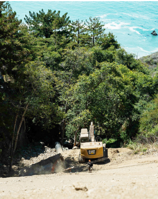
Working on such a precipitous incline required careful planning
