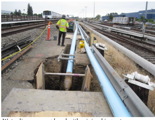
Water lines were replaced with minimal impact on BART operations
