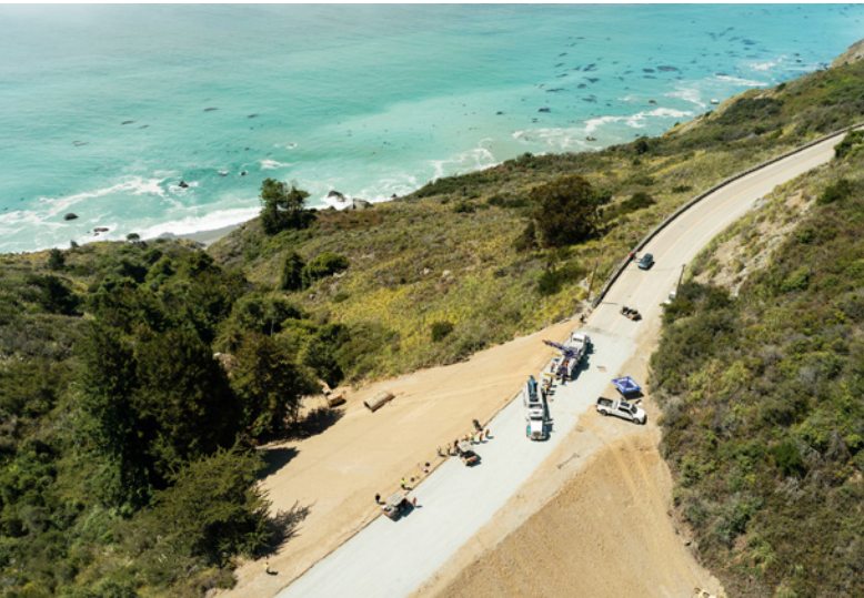
Project showcased public/private sector collaboration in completing complex infrastructure projects
