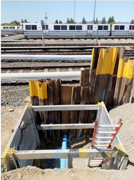
Many pipe bursting runs exceeded 600 feet under multiple BART tracks
