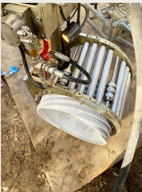
Winding machine spirals a PVC strip into the deteriorated pipeline
