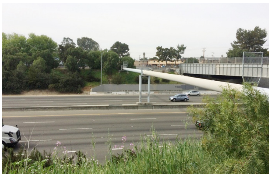
Figure 1. Photo of the 30-inch diameter high pressure natural gas line aerial crossing of I-880
