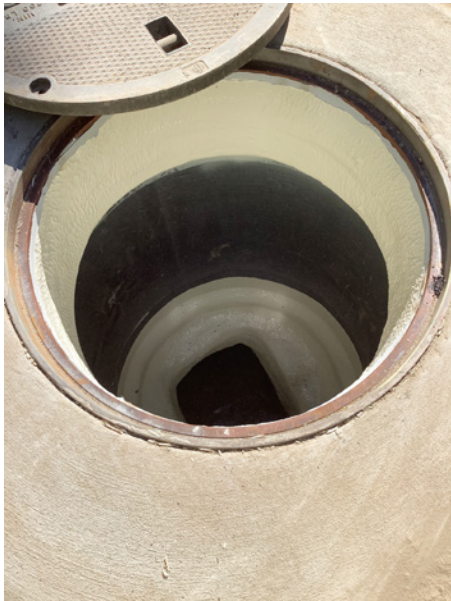
Manhole collar and bench coated with Zebbron
