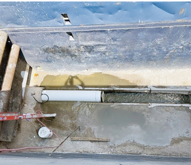
Insertion pit shown: A-2000™ PVC used to slipline the host pipe
