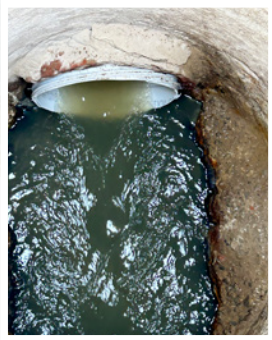
Liner is installed from the downstream to the upstream manhole
