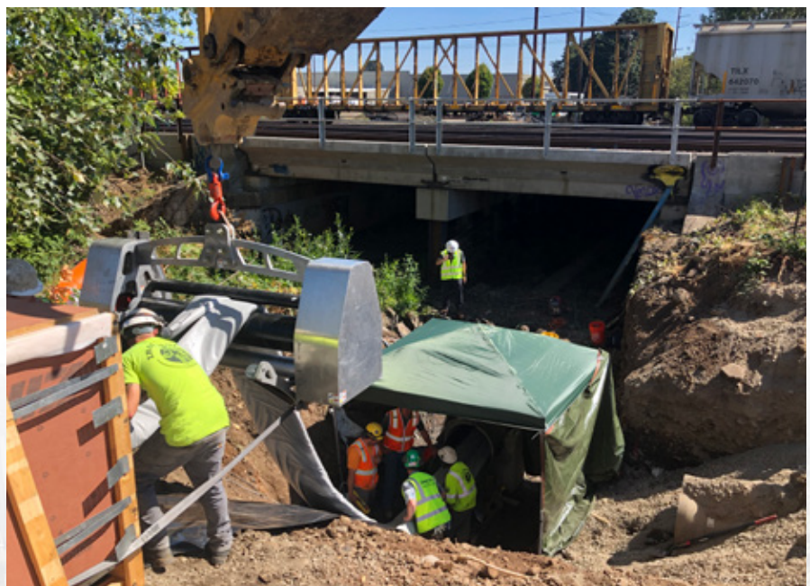
Liner Installation
