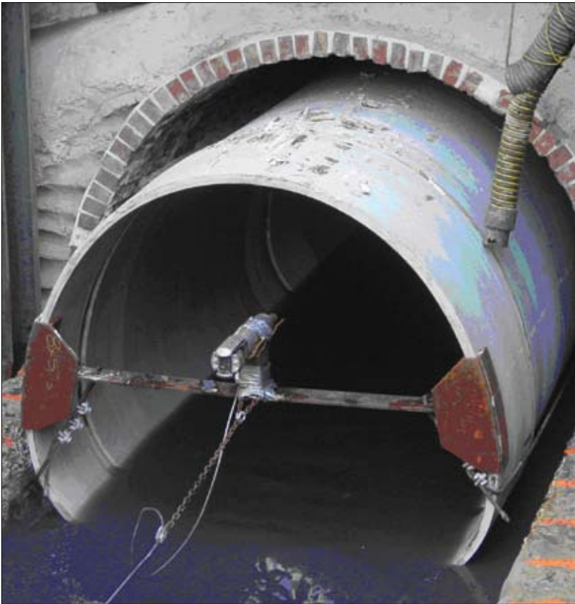
Figure 2. Installation of the 66-in. slipliner
