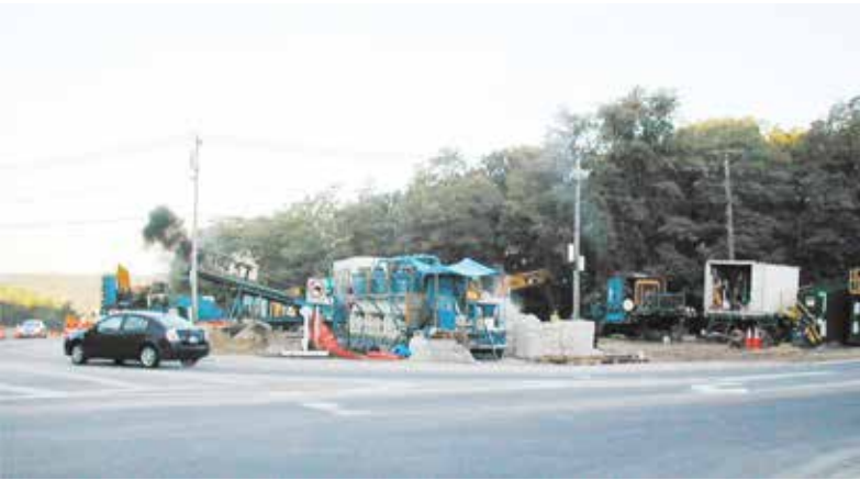
HDD can effectively protect delicate ecosystems while meeting societal and infrastructure needs
