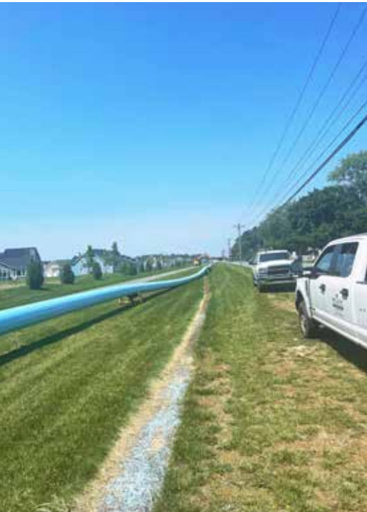
Figure 2. Melcar Preparing to Pull over 2,300 feet of 20-inch FPVC
