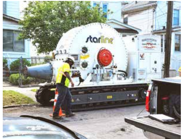
The Starline® Cured-in-Place-Lining Inversion Drum
