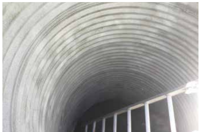
Figure 2. Riser pipe after it was media blasted and cleaned
