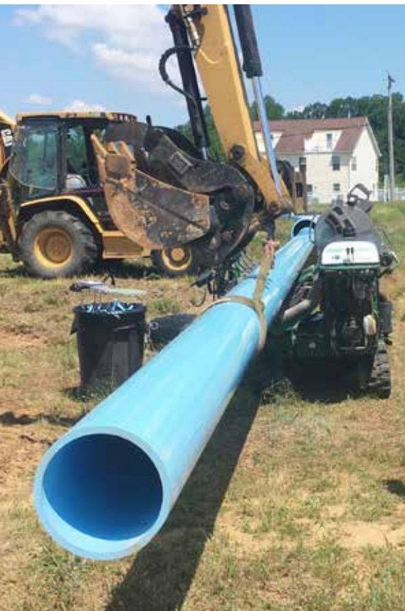
Figure 5. Spring Crew shown loading the 10-inch into 16-inch casing for pullback
