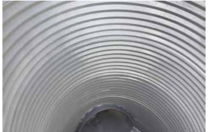
Figure 3. Riser structure pipe after OBIC Armor 1200C coatings
