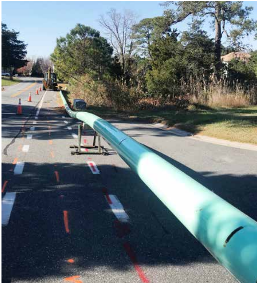
Figure 6. 10-inch Force Main ready to go at White's Landing
