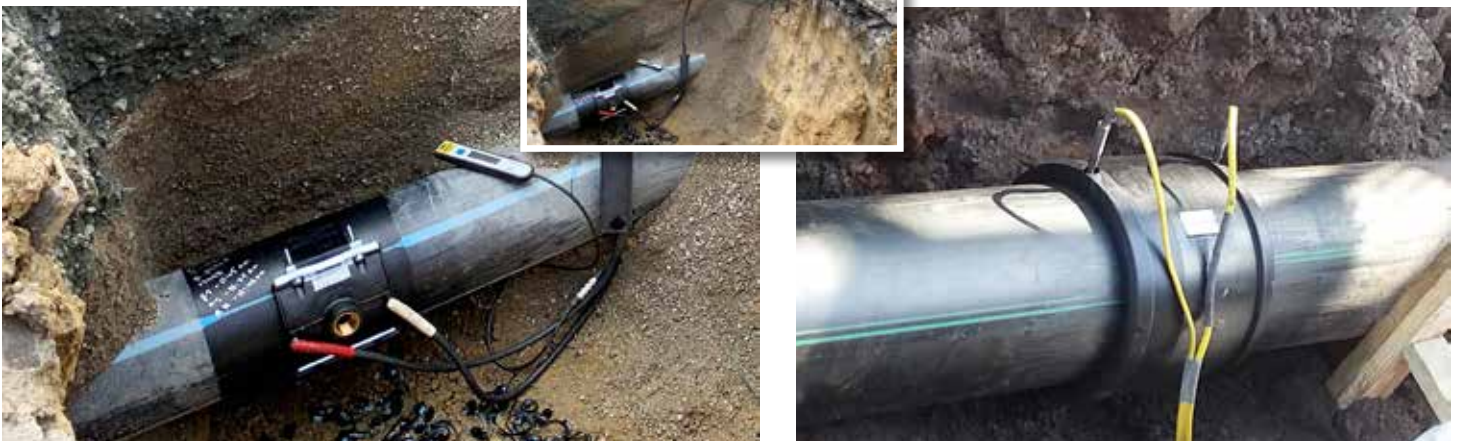
Electrofusion in Pit
