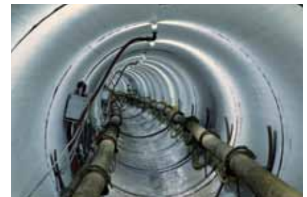
Figure 5. The completed curve with the tunnel support lines still in place.
