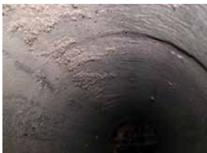
Figure 3. Image of the inner surface of the 26-year old, 6-ft long CIP liner section.
