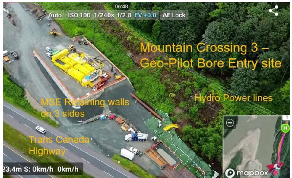
Figure 9. Mountain 3 Geo-Pilot Bore Entry Site with casing
