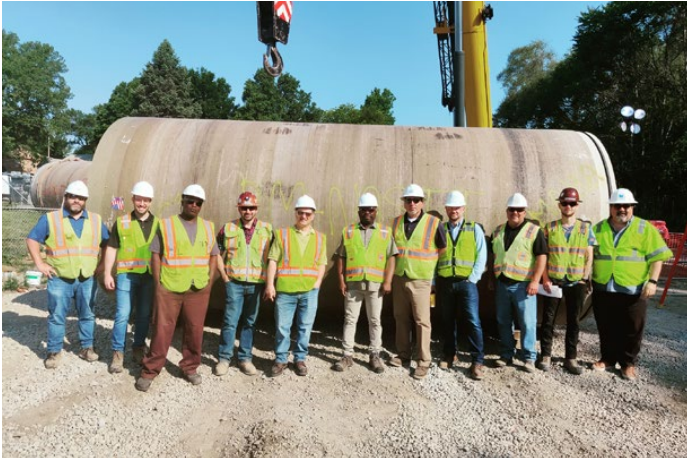
RMNASTT sponsored tour of the microtunnel construction
