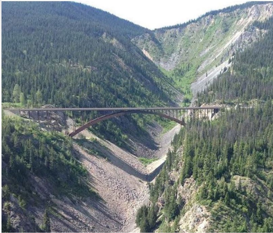
Figure 4. Dry Gulch at Highway and Pipeline Crossing
