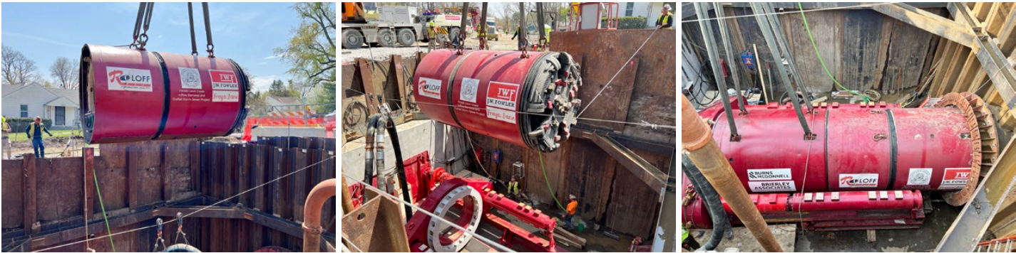
96-inch microtunnel crossing was successfully completed in June 2023
