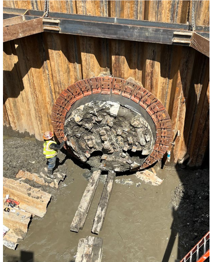
Successful completion of the trenchless crossing within project specifications
