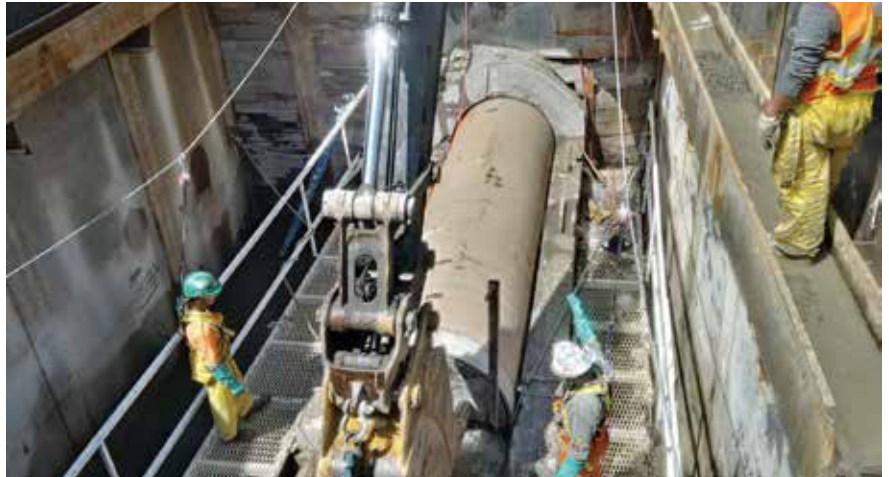
FIGURE 5: Shaft and Sliplining.
