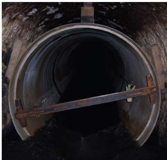
Figure 3: Sliplined pipe in place prior to grouting.
