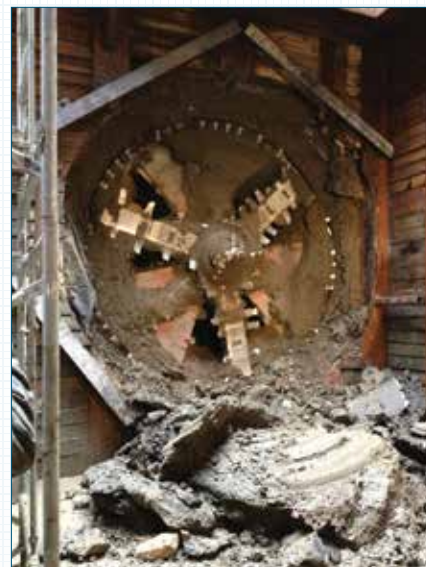
Figure 6 - 3,300-millimeter (130-in.) TBM breakthrough into reception shaft.
