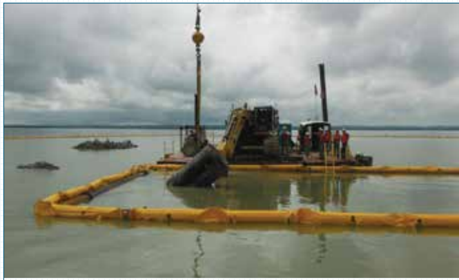
Figure 4 – MTBM being retrieved from the dredged trench.
