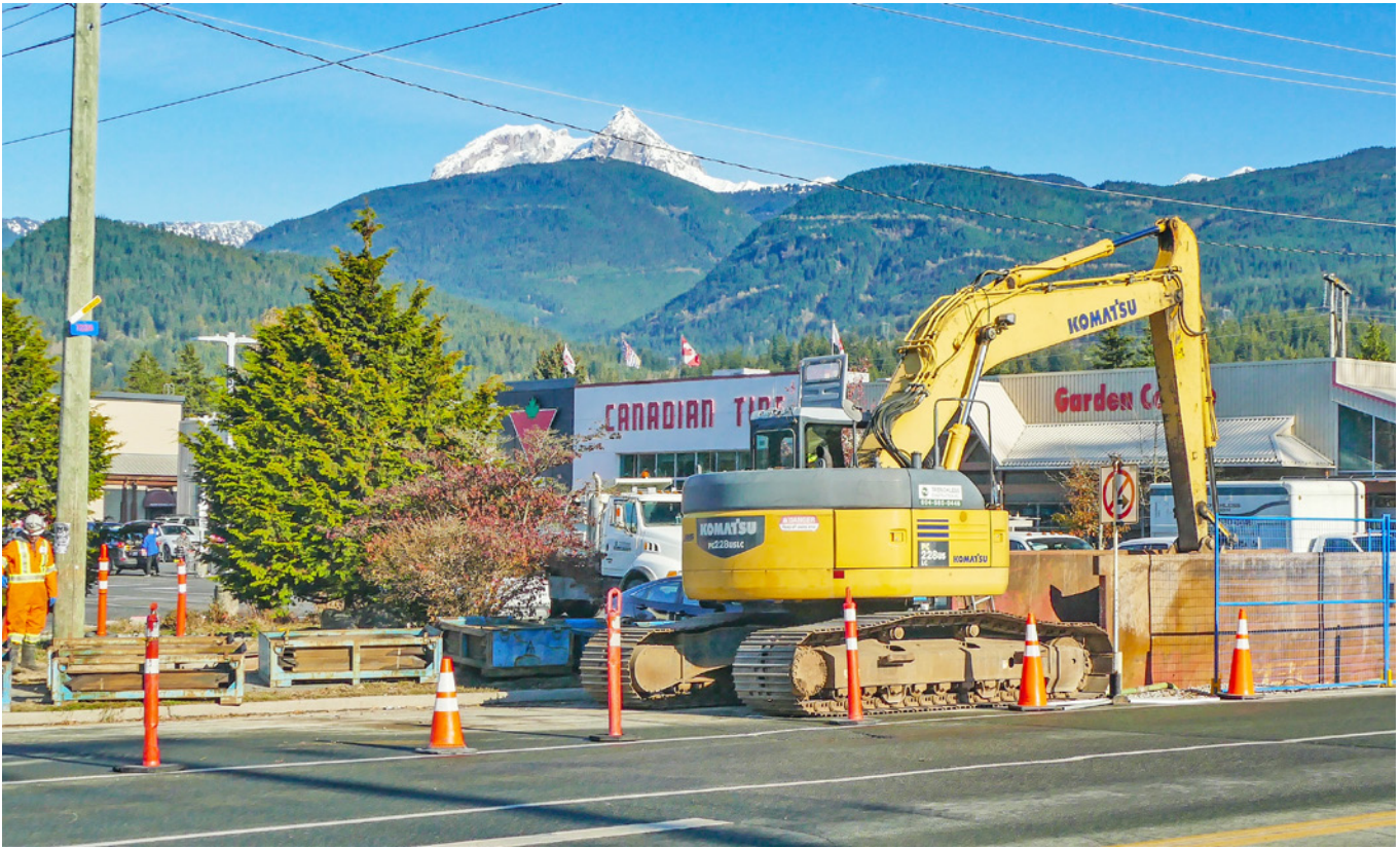
Complex project created minimal traffic disruption along busy highway
