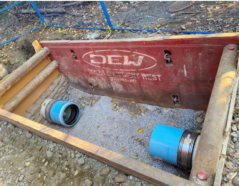
Lining completed and ready for the PWT crews to finish the connection
