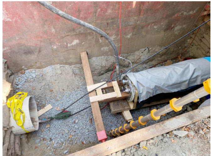
Set up for the UV light curing process
