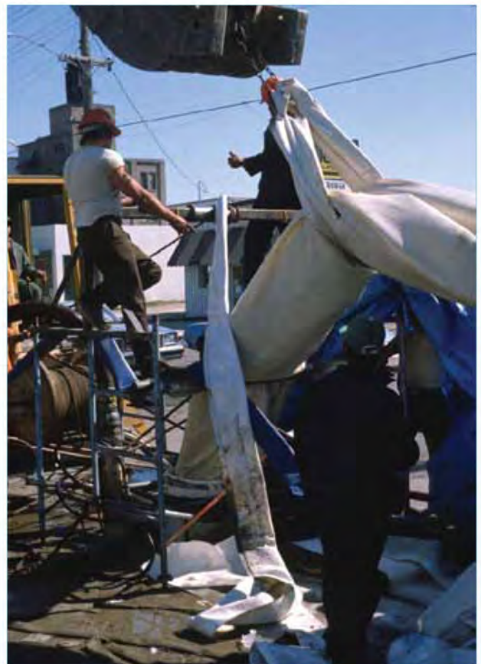
Figure 3: Installation of the Mission Secondary CIPP liner in April 1984.
