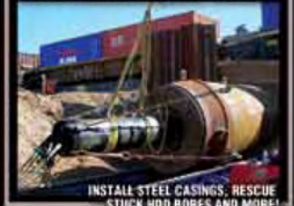
PIPE RAMMING/HDD ASSIST
